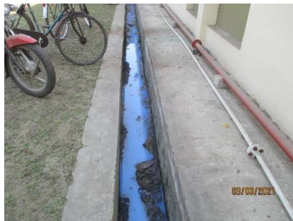
NC Photo # 10 Wastewater drained directly to drainage line
